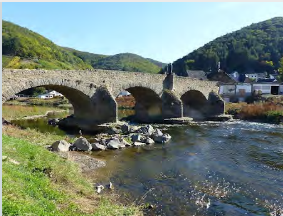
24 The Nepomuk Bridge in Rech
