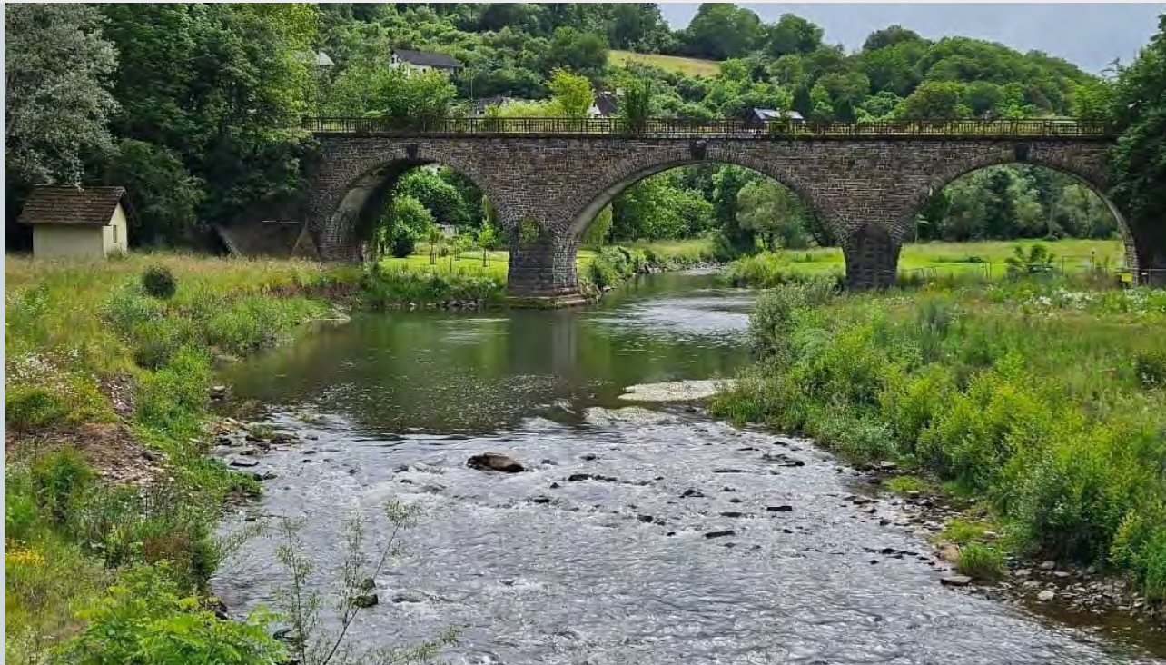
17 Railway bridge in Dümpelfeld
