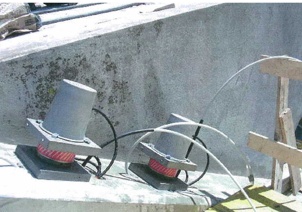
Abb. 7: Felsanker am Widerlager Nord, 2003
