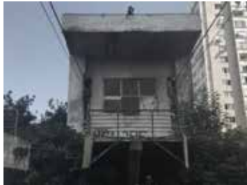
Fig. 10: IDP inhabited upper station in Vazisubani.
