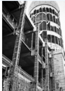
Figure 17: Steel Construction of the Tower Building (2024) © traveloutandish.com
