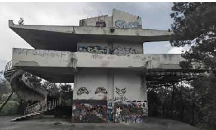
Fig. 12: Side View of the Upper Station
