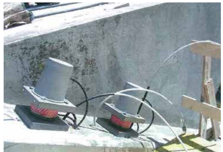
Abb. 7: Felsanker am Widerlager Nord, 2003
