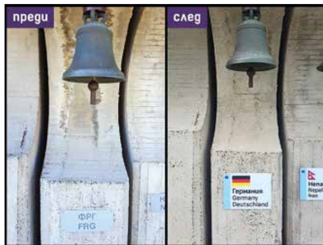
Fig. 12: Cleaning of the concrete semi-circles with bells, before and after sandblasting and labelling (Save Sofia archive)
