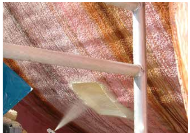
Fig. 6: Fresh foam being sprayed into the prepared voids (© adb Ewerien und Obermann)
