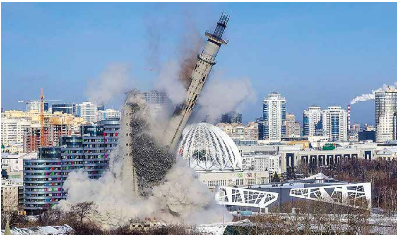
Fig. 4: The demolition ( http://www.brodyaga.com/pages/viewlarge.php?id=51040&cty=Ekaterinburg&place=Russia%20Sverdlovsk&region=Sverdlovsk )
