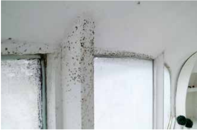
Fig. 12: Inside the deck before restoration (2015): frozen condensation on the windows, water and mould on the concrete shell (© adb Ewerien und Obermann)
