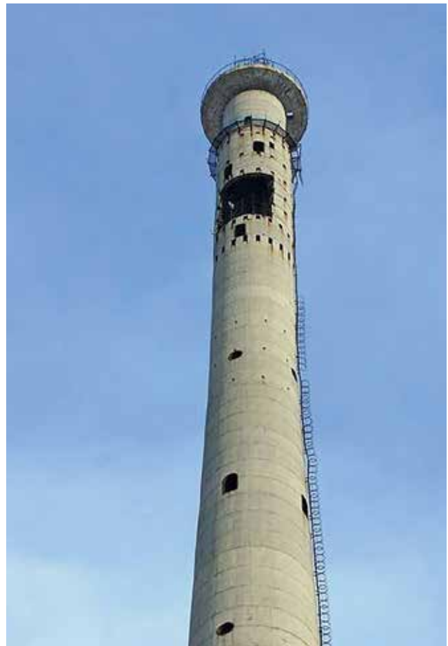
Fig. 3: The TV tower before demolition ( https://neferjournal.livejournal.com/4710982.html )
