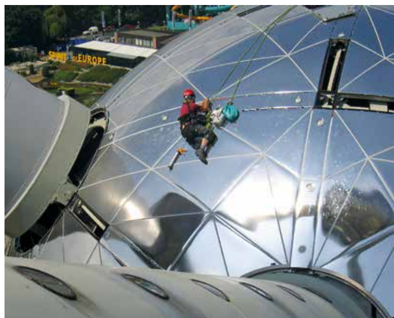
Fig. 6: Installing the meridian plates (photo Origin 2005)
