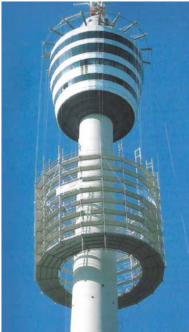
Fig. 9: Elevator on ropes for external repairs
