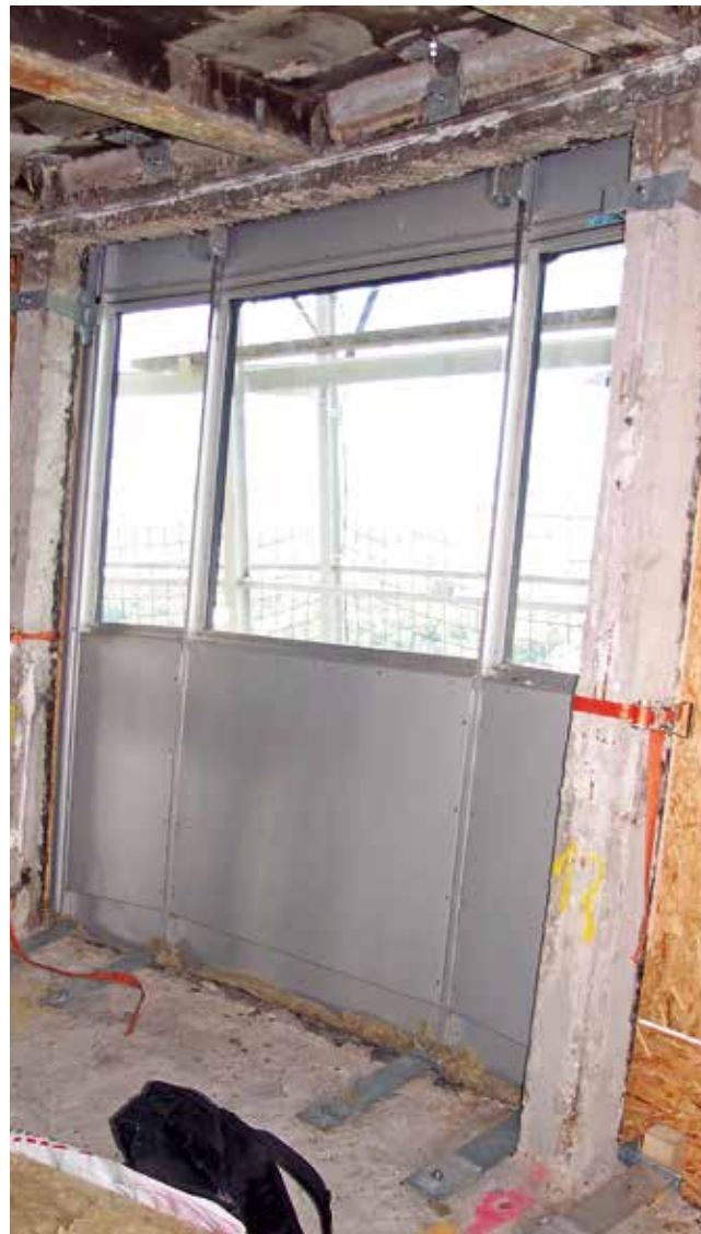
Fig. 10: Replacement of facade elements
